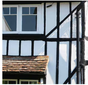
Half timbering with render or brick infilling
