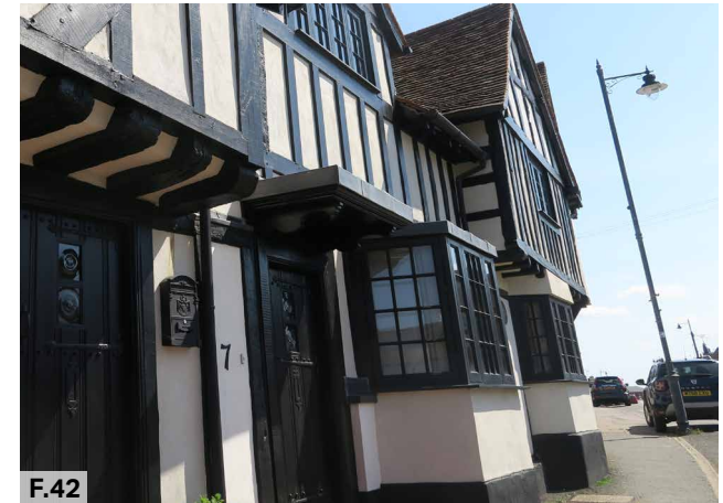
Figure 42: Detail of a ground floor with restored multi-pane bay windows
