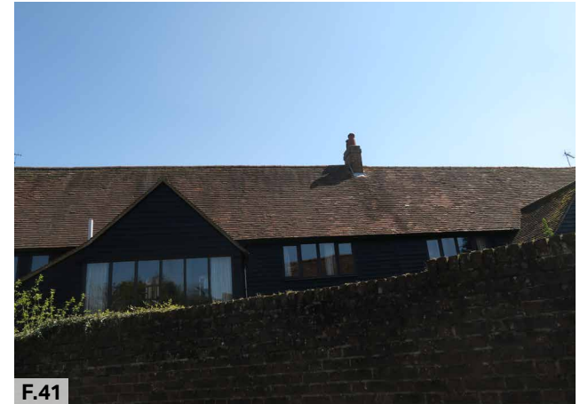
Figure 41: A building with traditional materials such as black weatherboarding and clay tiles
