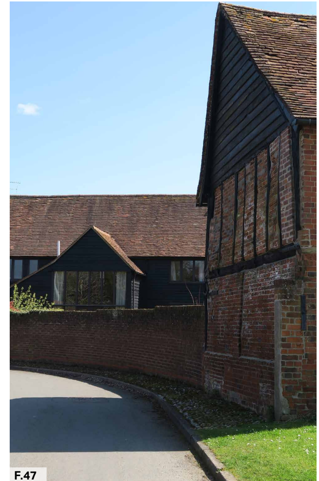
Figure 47: Agricultural buildings with weatherboarded gables and red brick boundary walls
