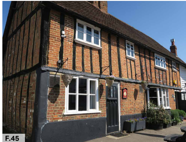
Figure 45: Listed building with half-timbered structure and red brick infilling
