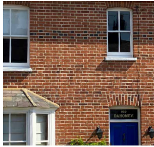
Red bricks in Flemish bond
