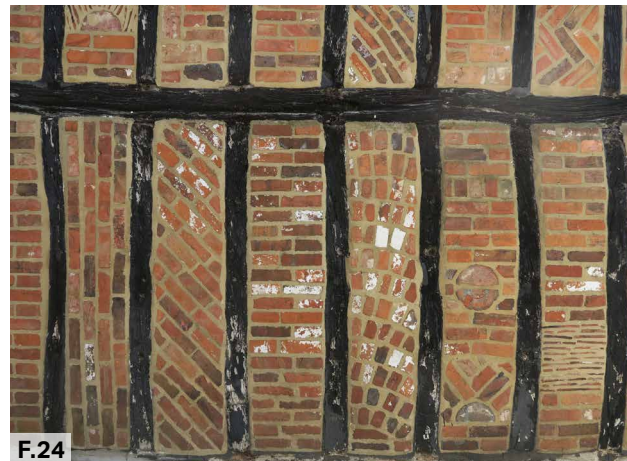
Figure 24: Half-timbered wall with different patterns of brick infilling
