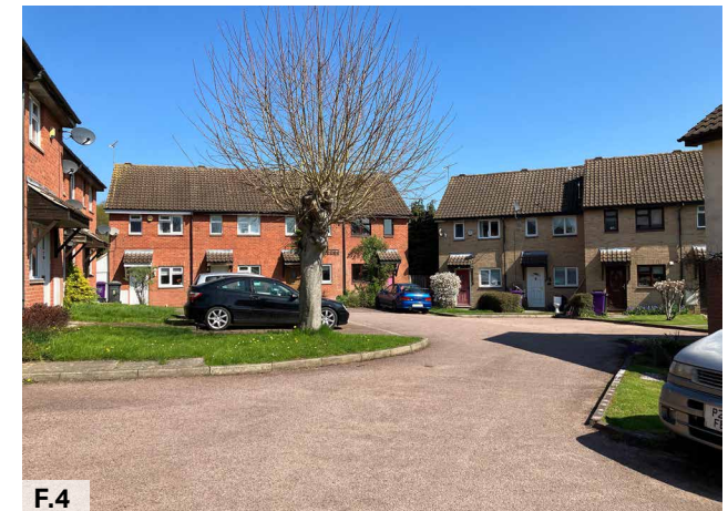
Figure 04: 20th-century terraced houses arranged around a cul-de-sac road
