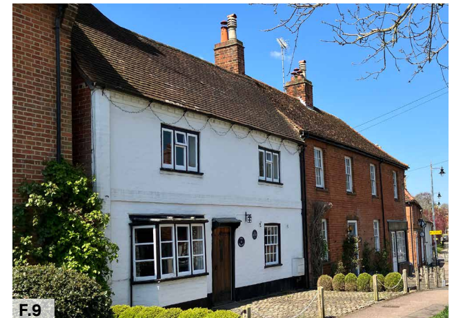
Figure 09: Grade II listed former Red Lion PH, now a house called The Noggins, with 17th Century timber frame, painted brick façade and dentilled eaves (source: Codicote Parish Council)
