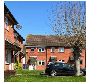
Pentice canopy porch
