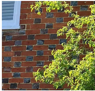
Checked bricks in Flemish bond
