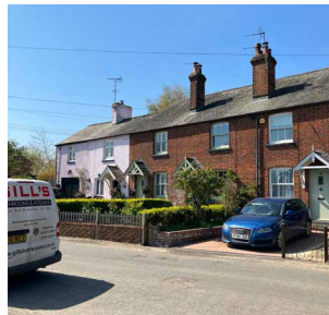
Pitched roof canopy porch
