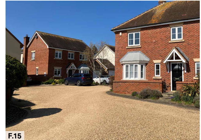
Figure 15: Parking courtyard with porous gravel surfacing on Dollimore Close
